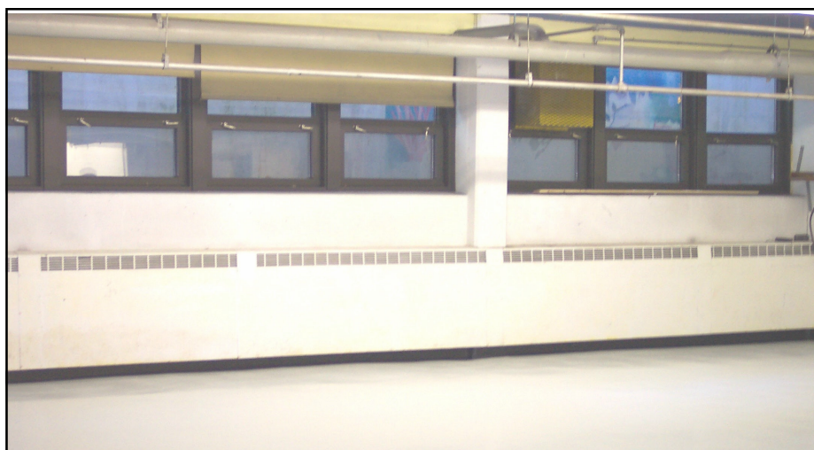
The auditorium basement has a clean new look since the disaster recovery team, Belfor, disinfected and cleaned it after the July flood.
